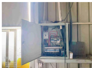
Electrical box without inner cover.jpg
